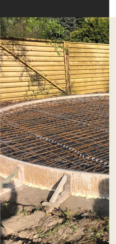
The tank is founded on a flat foundation slab made according to JRtech guidelines. The basic scope of the foundation slab design includes:
